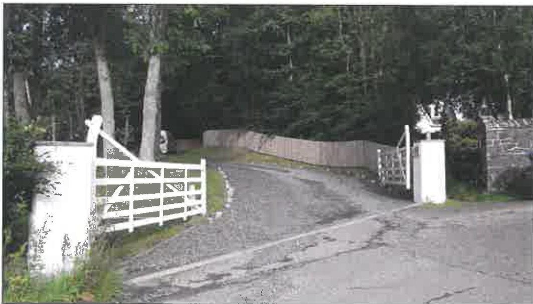
Fig 6: Access into Craigerne Coach House which will be used by the plot
